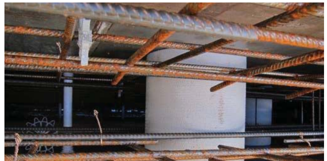
ZVR 200/300 fixed in formwork
