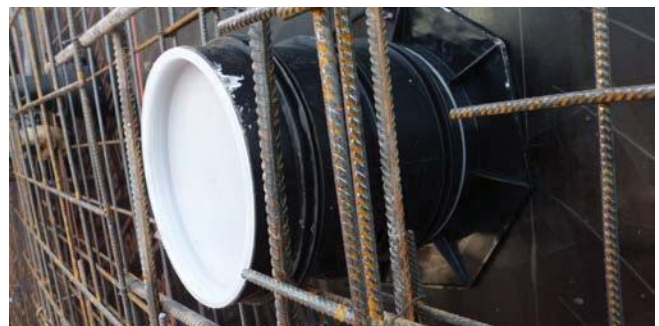
UFR in formwork
