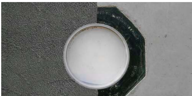
concreted UFR with PMBC
