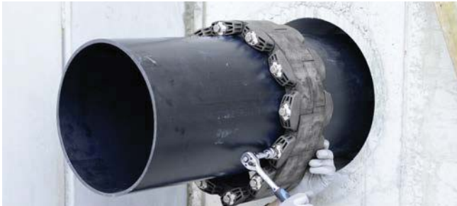
GKD 400 – tightening of segments
