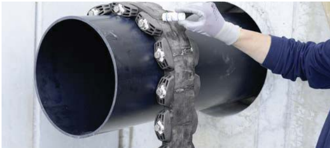
GKD 400 – installation preparation with lubricant GM
